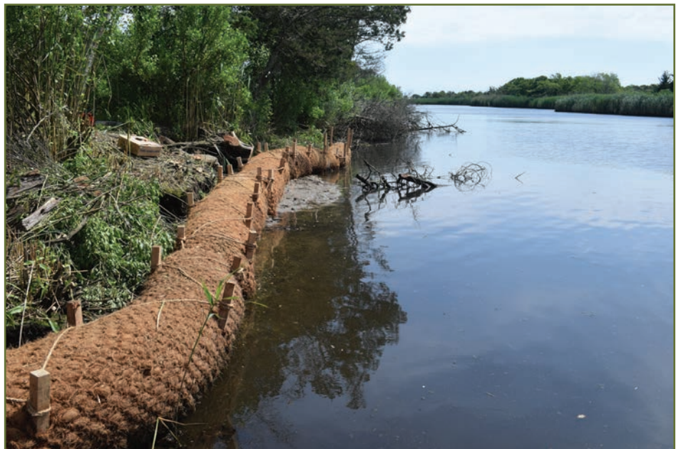
Coir logs installed along the edge of Beaver Dam Creek next to the boardwalk for erosion control.
