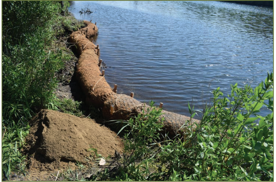
Coir logs installed along the edge of Beaver Dam Creek next to the boardwalk for erosion control.
