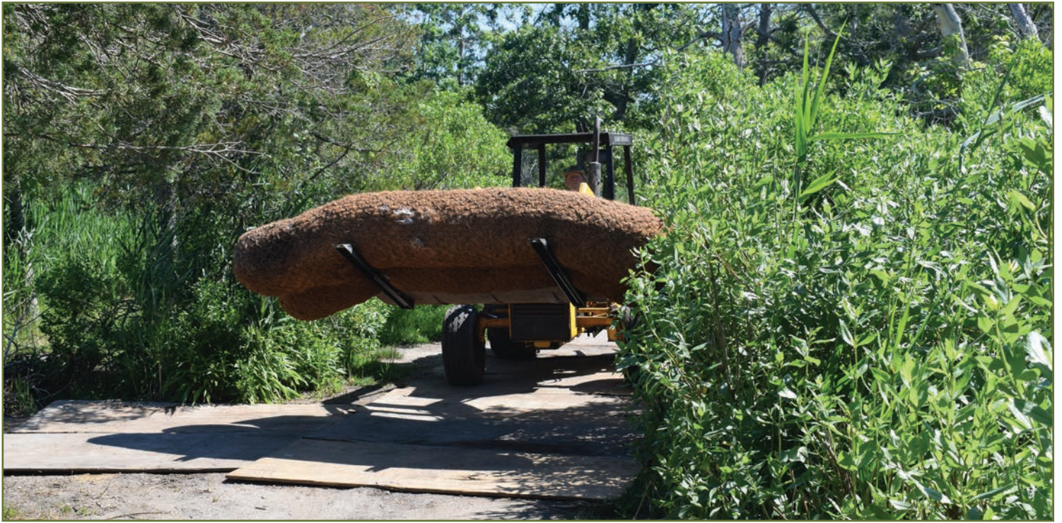
Coir logs from the Wertheim Refuge being delivered to the site.
