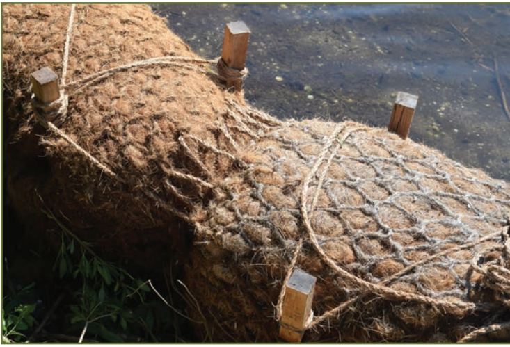
Coir logs tied together and staked into the creek edge.
