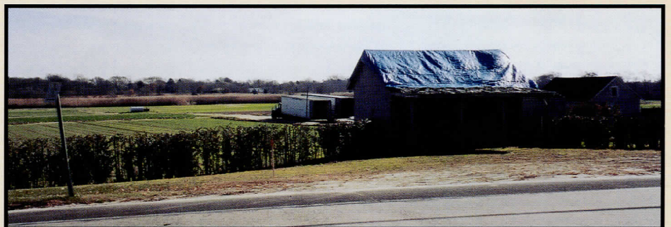
The farmstand undergoing renovation in anticipation of this summer's opening
